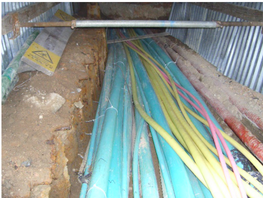
Photo 4 - 22kV Cables
