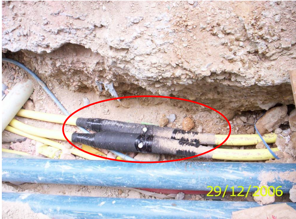
Photo 13 – Pilot Cable Joints
