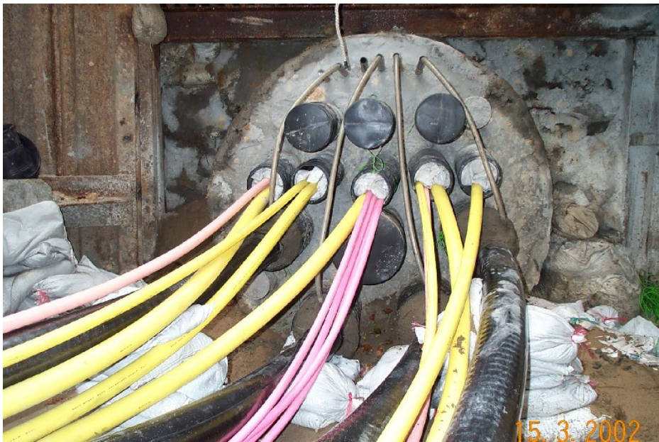
Photo 8 – 132kV Cable Ducts
