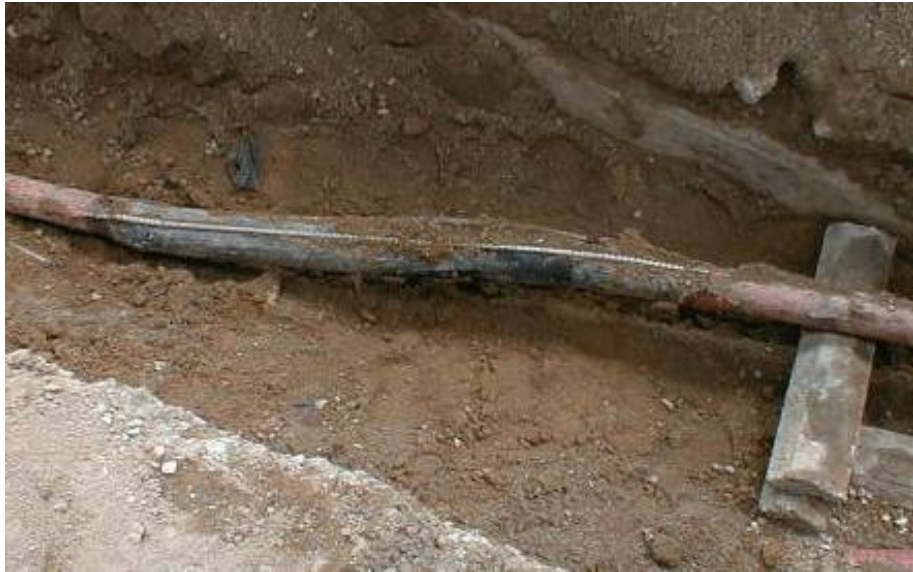
Photo 3 - 11kV Cable Joint
