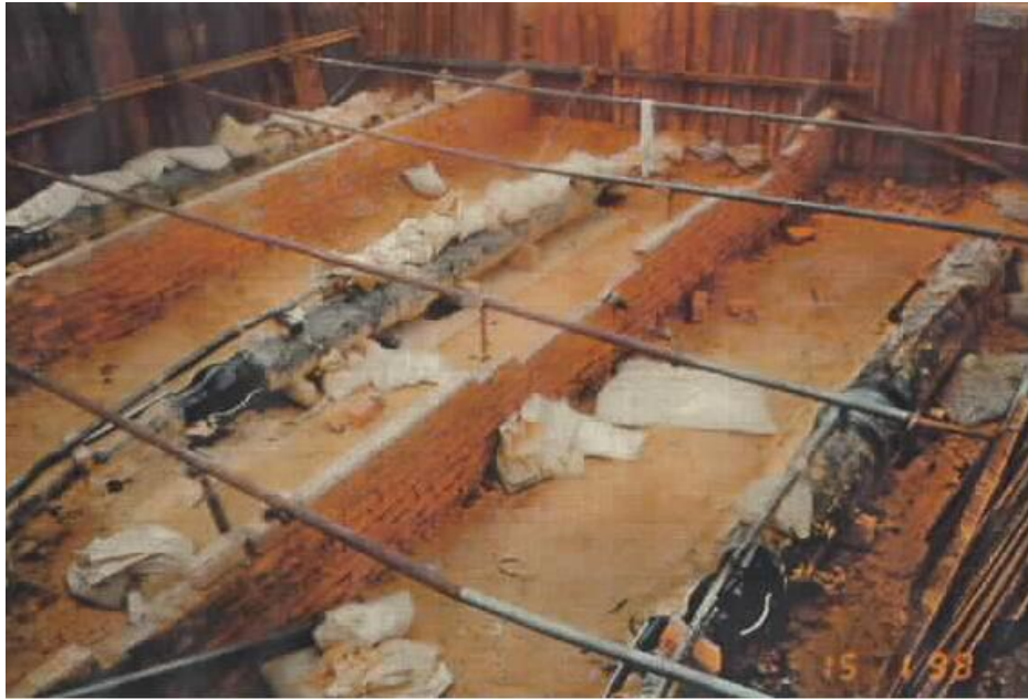
Photo 11 – 275kV Cable Joints
