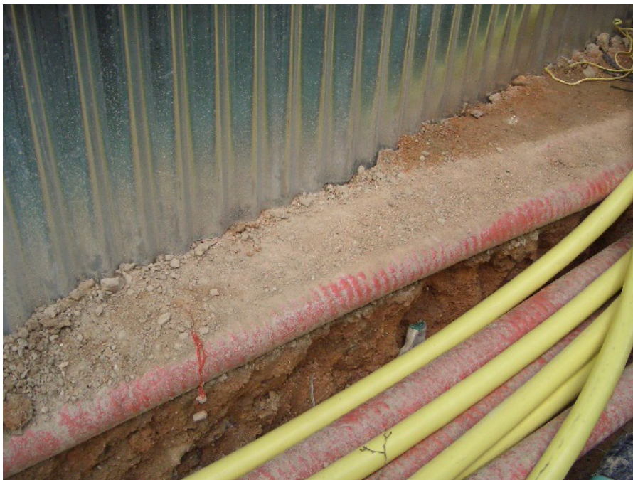
Photo 2 - 11kV Cables
