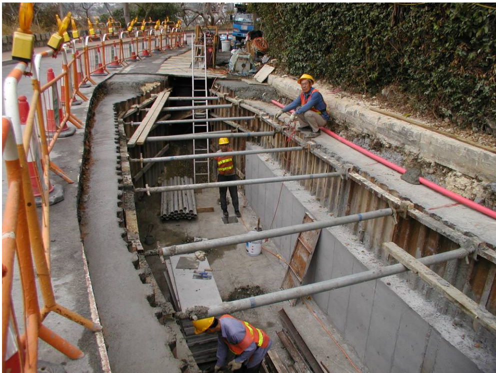
Photo 20 – Transmission Cable Joint Bay
