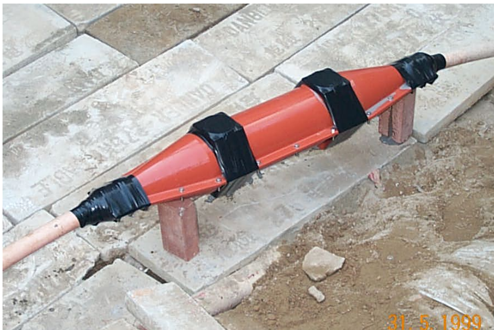
Photo 14 – Optical Cable Joints
