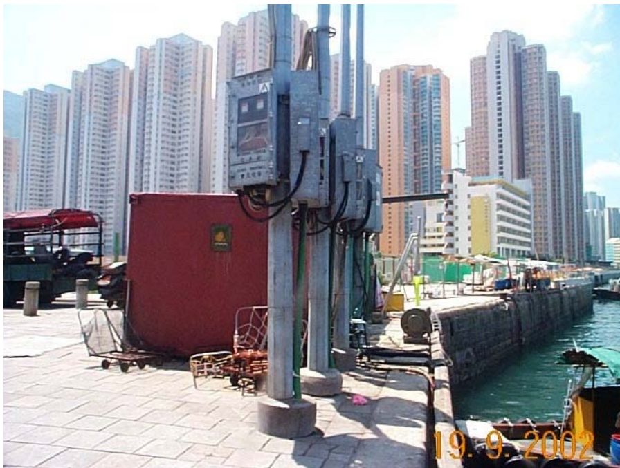
Photo 16 – LV Overhead Line Poles
