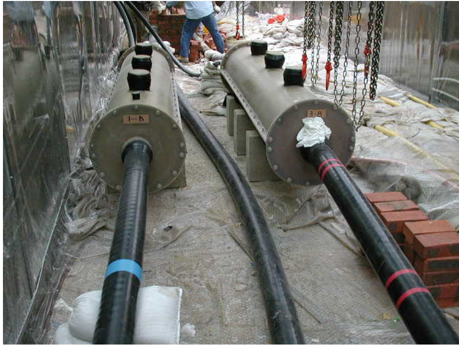
Photo 9 – 132kV Cable Joints
