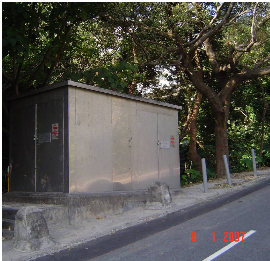
Photo 17 – Transformer Pillar
