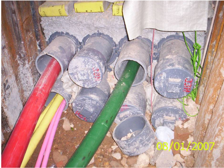
Photo 5 - 11kV, LV and Communication Cable Ducts
