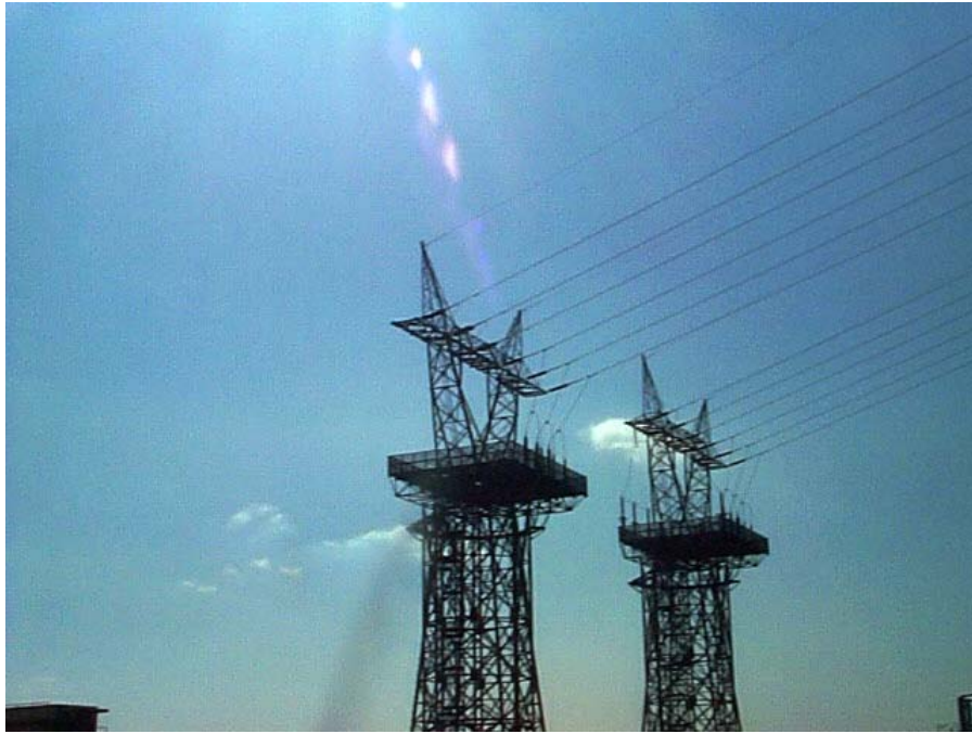
Photo 15 – 132kV Overhead Line Towers
